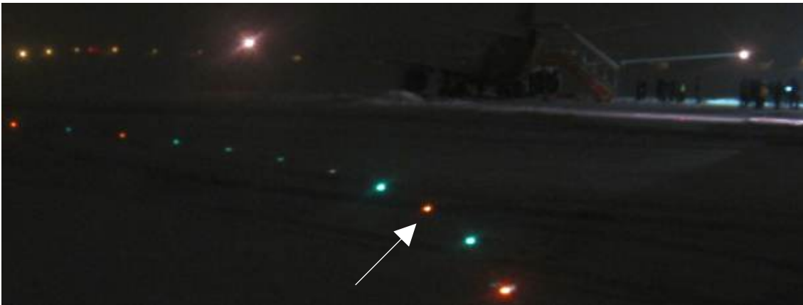
[Figure 3] Runway and Taxiway Centerline Lights
