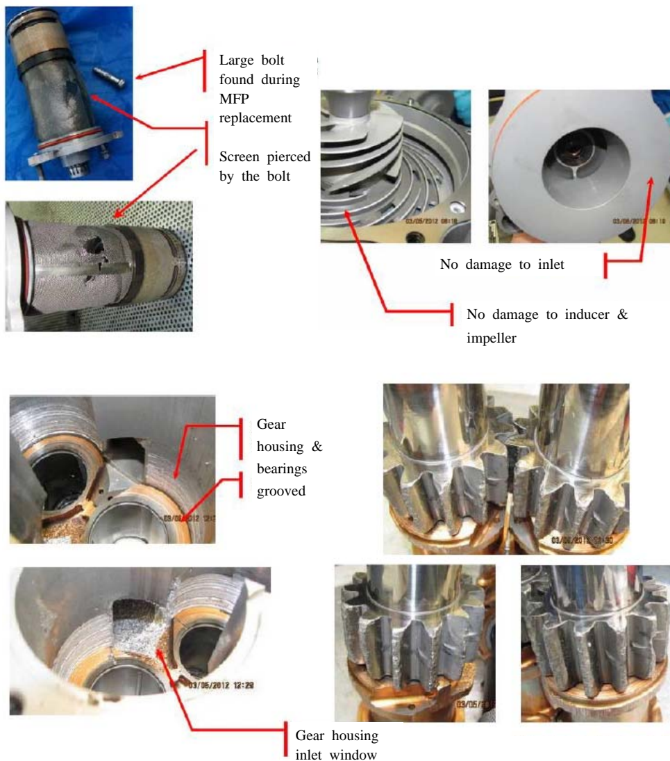
[Figure 9] Inspection of the Fuel Pump
