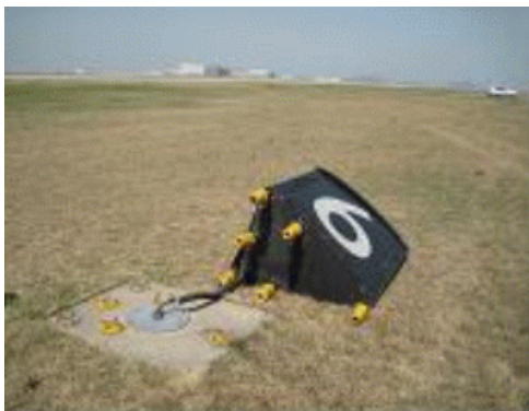
[Photo 6] Runway distance marker sign damaged
