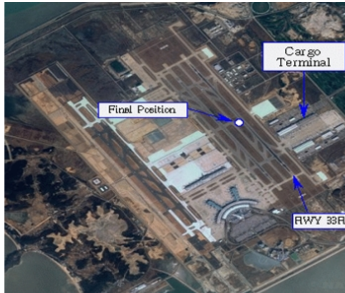
[Photo 1] General view of the Incheon Airport runways
