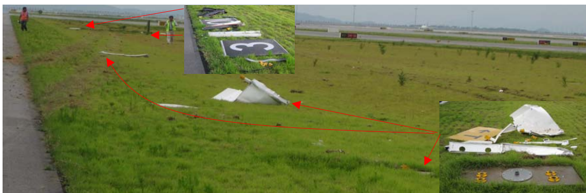
[Photo 8] Runway distance marker sign damaged
