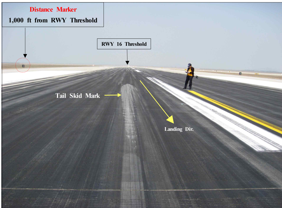
[Figure 7] Tail Skid Mark on Runway
