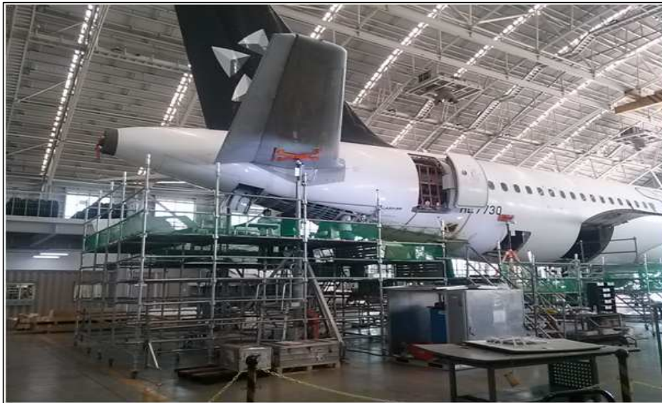
[Figure 4] Aircraft Repair
