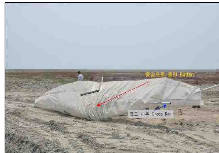
[Figure 14] Accident Site
